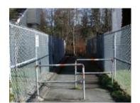
Generally, use metal bollards in more urban environments, and wood bollards in more natural settings or where a wood fence or railing is used at a trail head.
