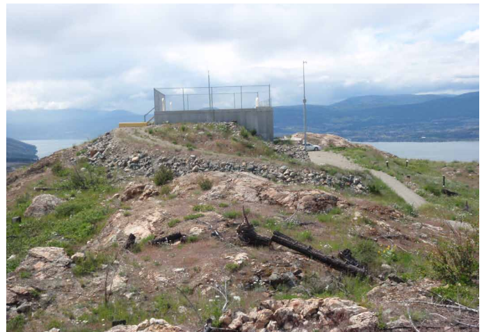
Kuipers Peak Reservoir - The location of this reservoir has a significant negative visual impact. Locating the reservoir behind the crest of the hill could have largely hidden the utility from public view.
