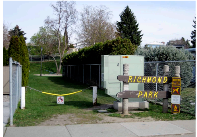
Richmond Neighbourhood Park - Above ground utility boxes on park sites can be unsightly and block sightlines into parks. Underground utility boxes are a preferable option.
