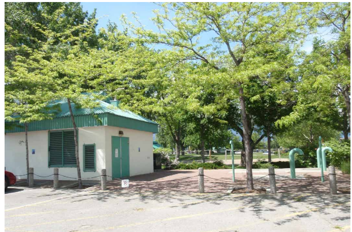
Gyro Park - The lift station at this park is located at one of the main access points to the park. It blocks views to the park, consumes park space, and impacts design attempts to create a welcoming park atmosphere.
