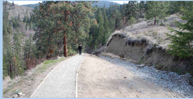
This hillside trail accommodates a rock fall area as well as a clear drainage course to maintain trail stability over time.
