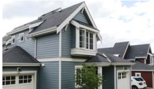
View of strata coach house units from laneway (photo: Michael Geller)
