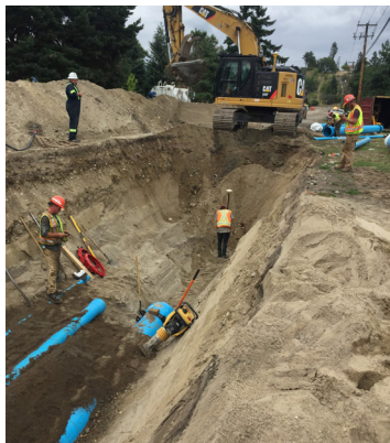
Above: Tie-in at Stellar Rd. pump station
