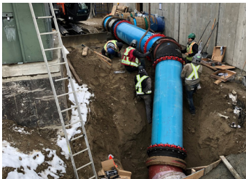
Above: Tie-in at Stellar Rd. pump station
