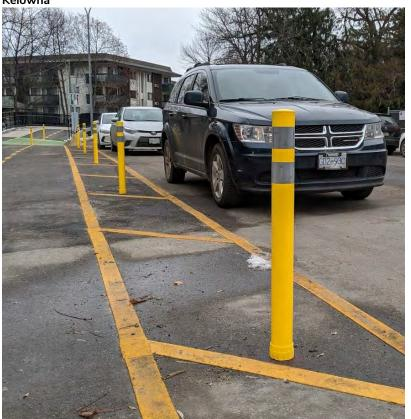
Figure 6. Protected bike lane using flexible delineator posts and on-street parking along Sutherland Ave in Kelowna
