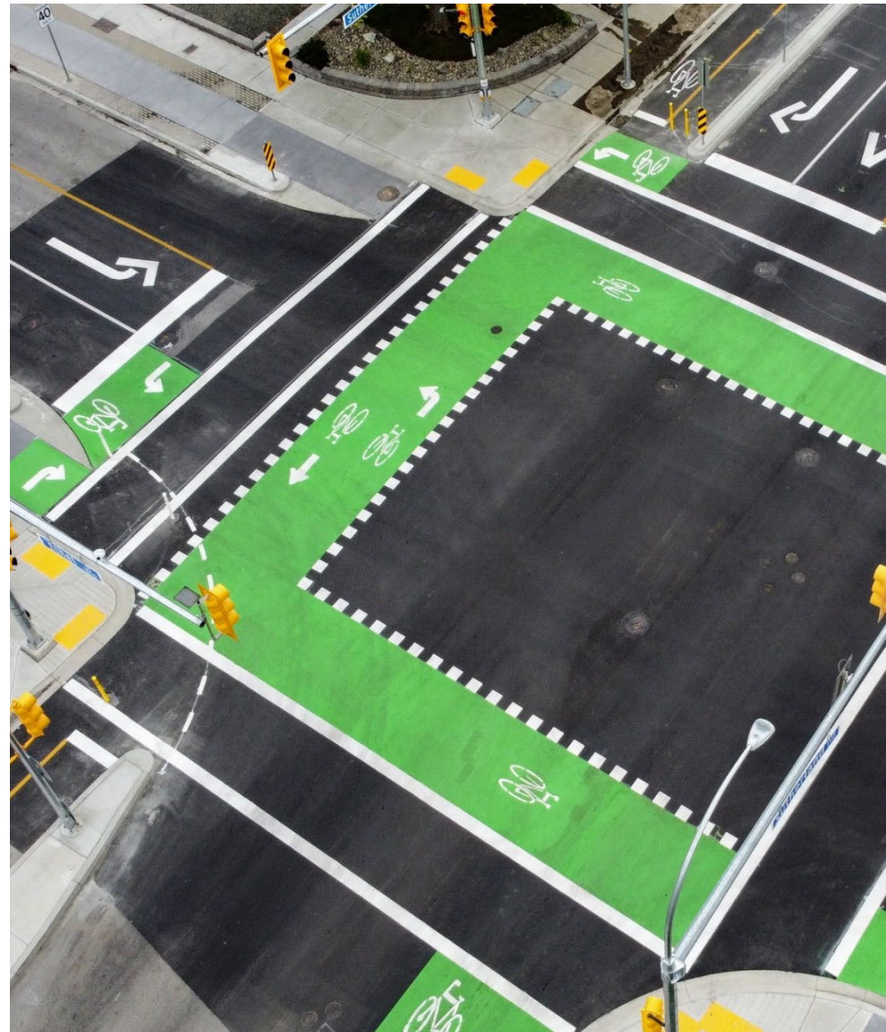
Figure 4 Intersection of Ethel and Sutherland in Kelowna where two protected bike lanes meet.
